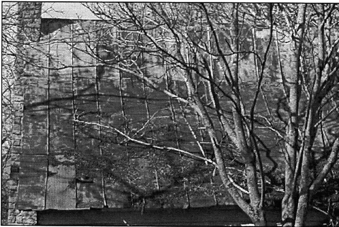
Photo #3: Rear slope of roof, note raised seam metal roof in fair to poor condition.
