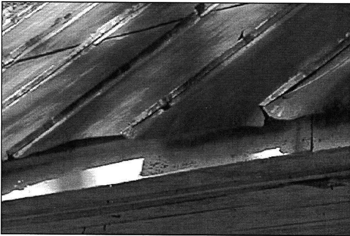
Photo #5: Detail of above, note seams not crimped; deteriorated condition of roofing.
