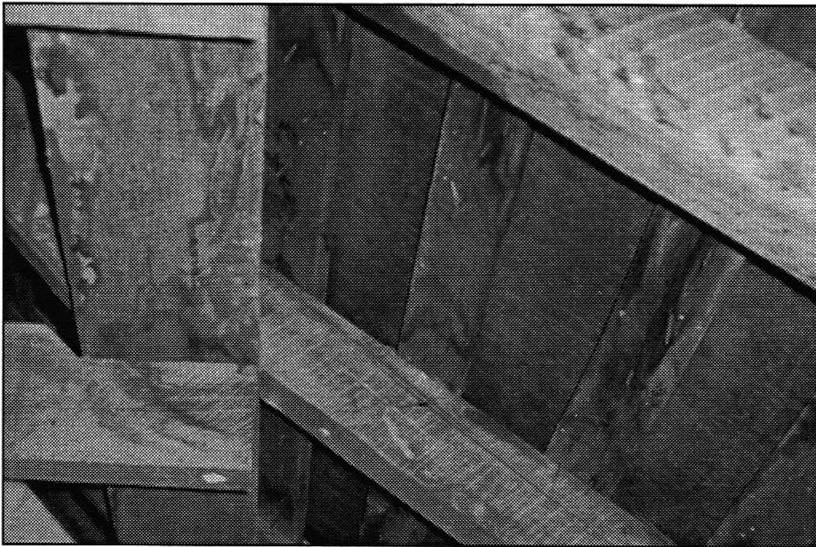
Photo #6: Interior at rear ell, note nails from older wood shingles protruding through roof boards.
