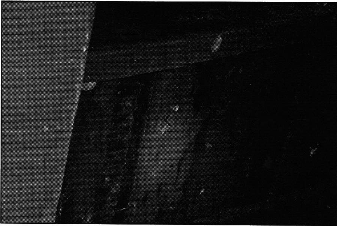
Photo #8: Interior at rear ell, note nails from older wood shingles protruding through roof boards.
