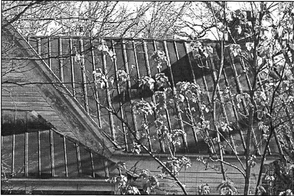
Photo #2: Front slope of roof, note V-crimped metal roofing in fair to poor condition.
